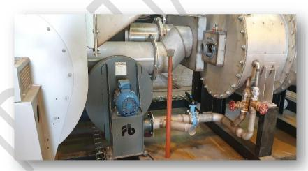
the gas burner to be mounted and also has a number of ports and instruments included to allow the syngas to be recirculated along with the supply of combustion air.
